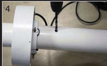
4 Drill a 0.4 inch hole under the unit
